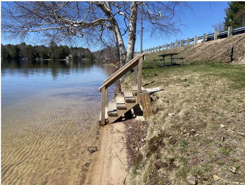
Figure 4: Existing stair access to water.
