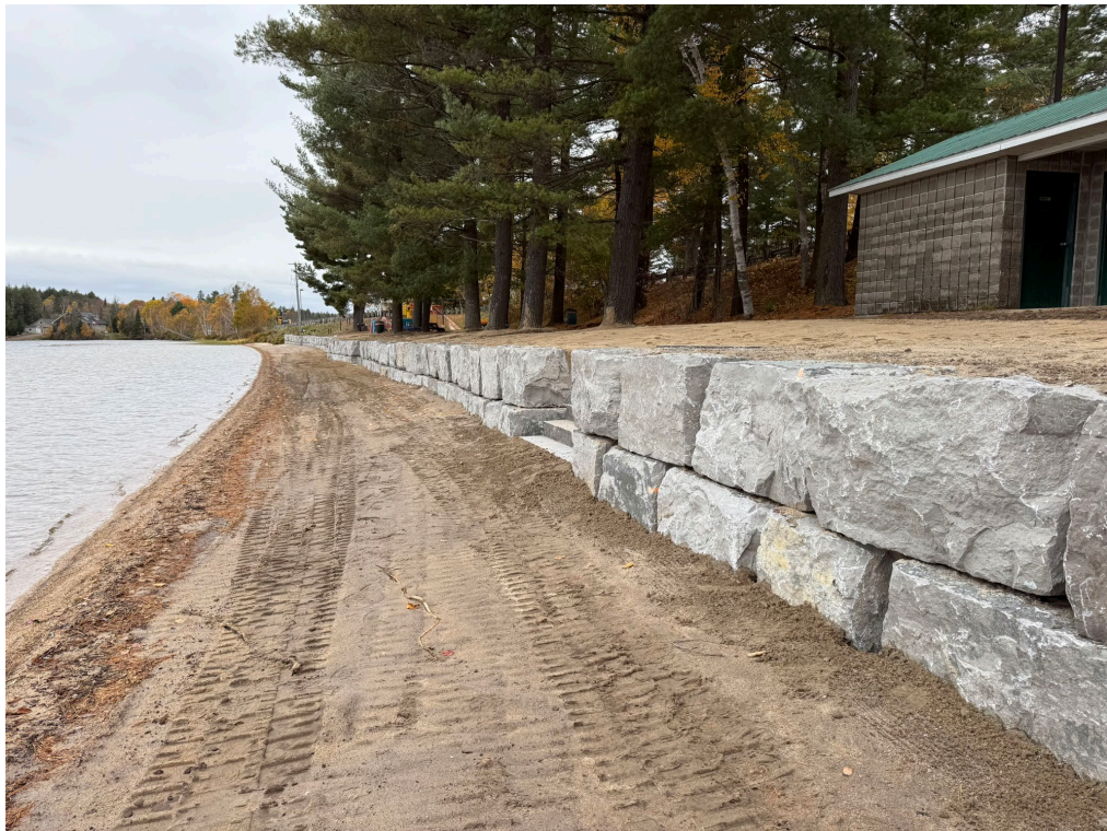
Figure 4: Constructed armour stone shore wall.
