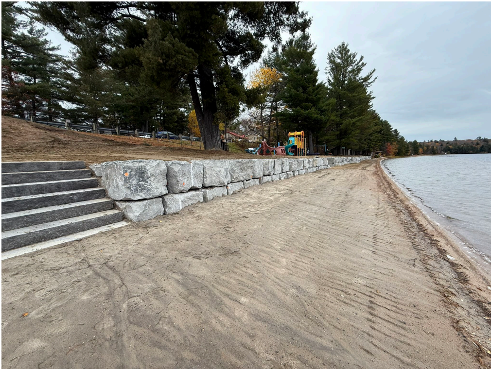
Figure 6: Stone step access to beach.
