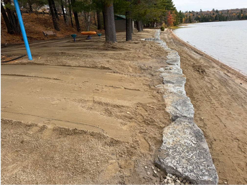
Figure 5: Minor adjustment to wall alignment to accommodate tree root systems.
