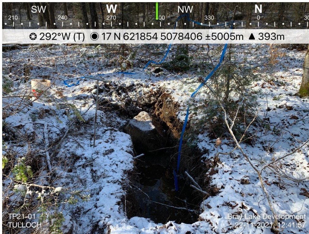
Photo 1: TP21-01 Excavated from previous investigation – standing water in bottom of test pit.
